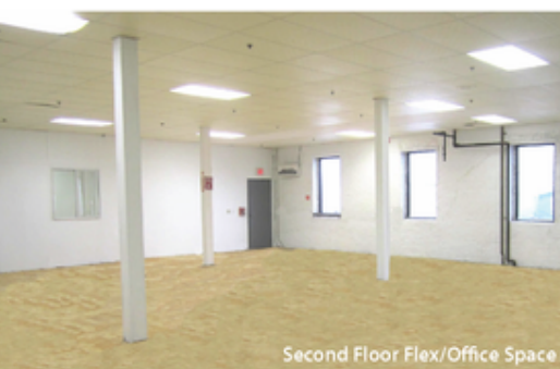
Second Floor Flex/Office Space
